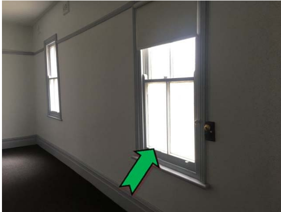
Photo 7. Interior, throughout, windows and window frames – non asbestos-containing window caulking.
