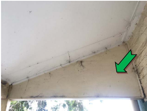
Photo 3. Exterior, entrance verandah, upstand panel – non asbestos-containing fibre cement sheeting.
