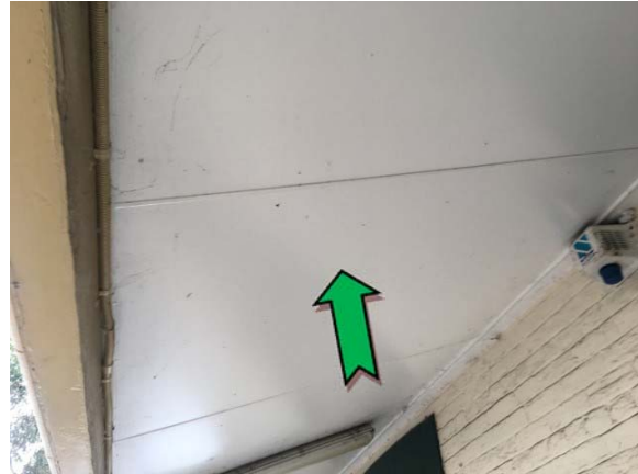
Photo 2. Exterior, entrance verandah, awning – non asbestos-containing fibre cement sheeting.
