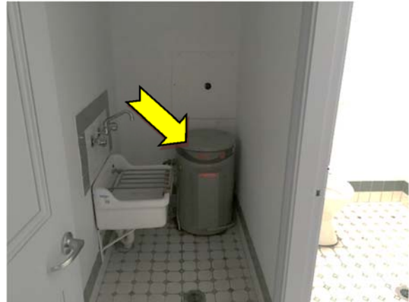
Photo 8. Interior, toilet, hot water heater – suspected SMF internal insulation material.
